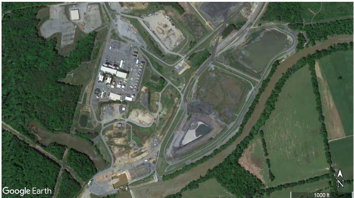
Overhead view of ash pits at the Dan River Steam Station. Image: ©2018 Google
