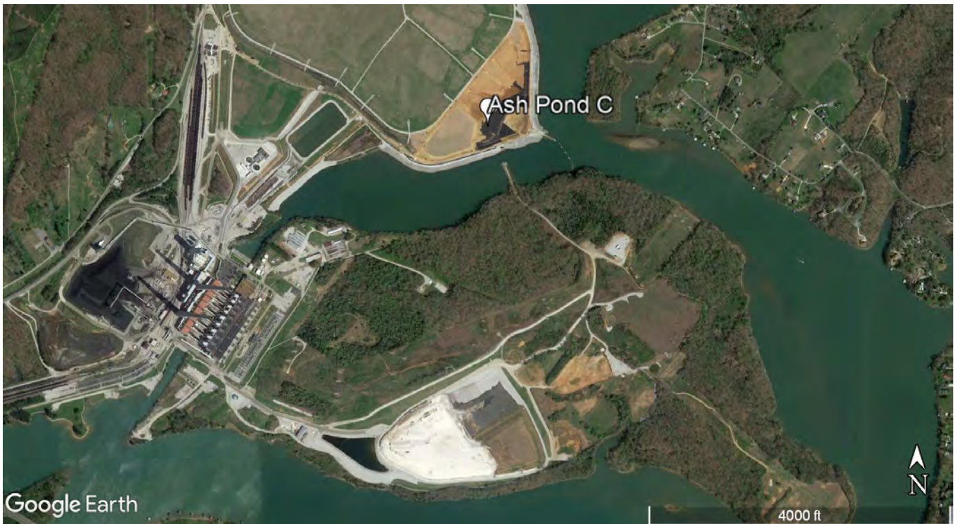
At the Kingston Fossil Plant, Ash Pond C contained decades worth of toxic coal ash waste. When the coal ash pit’s dike failed, more than 1 billion gallons of coal ash waste flowed into the nearby Emory and Clinch rivers. 28 Image: ©2019 Google
