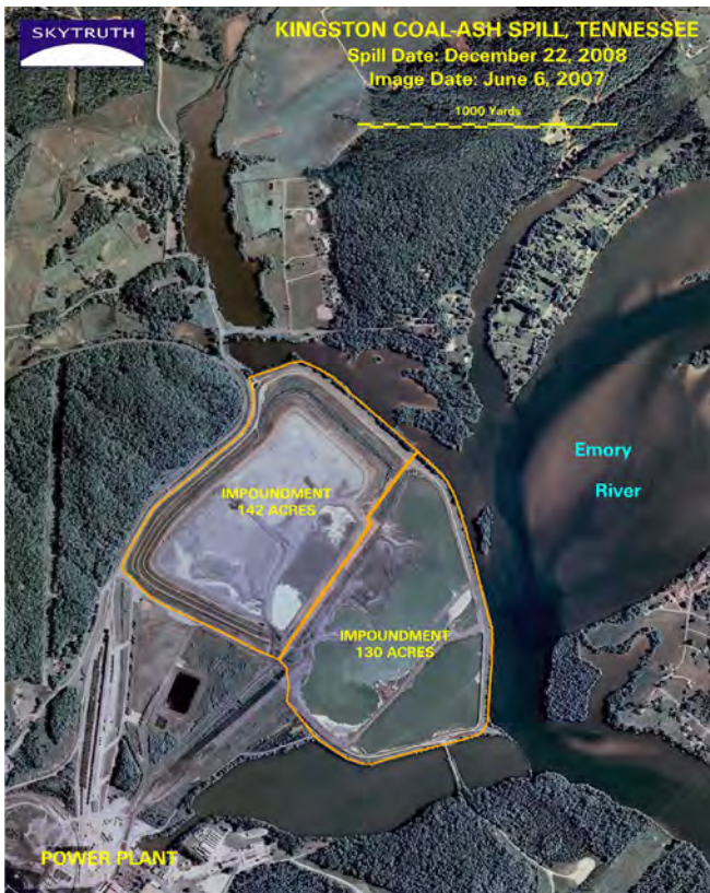
Often, coal ash pits are separated from water by only a thin retaining wall, as was the case for a pit at the Kingston Fossil Plant in Tennessee, the site of one major spill. Image: Skytruth via Flickr (CC BY-NC-SA 2.0)
